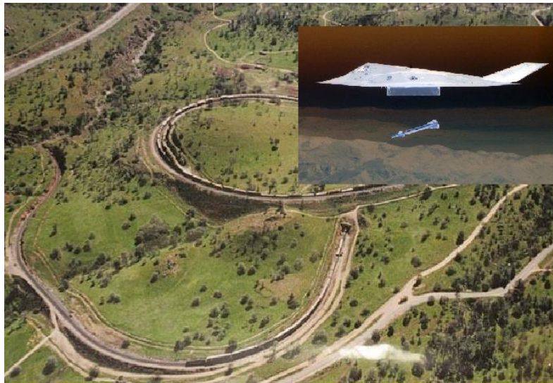
Figure 136. Railway section to be destroyed.
