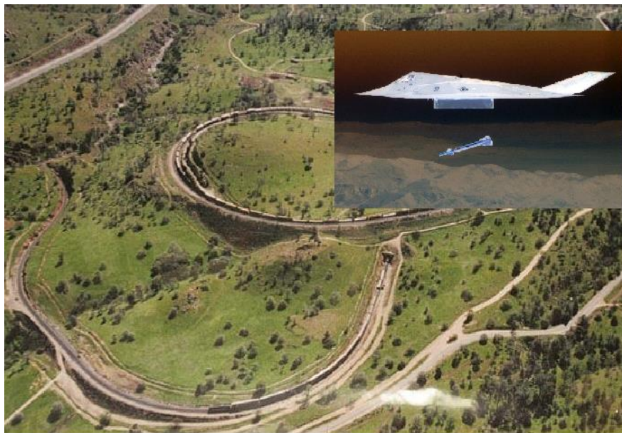
Figure 137. Railway section to be destroyed
